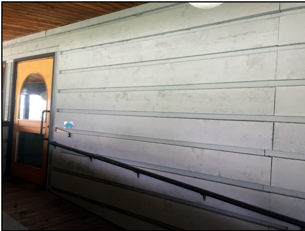
Photo 12: The doorway located at the top of the ramp on the east elevation; the position of the original main entrance is apparent where several courses of siding align at butt joints (Cultural Alaska/Wellspring Group 2017).
