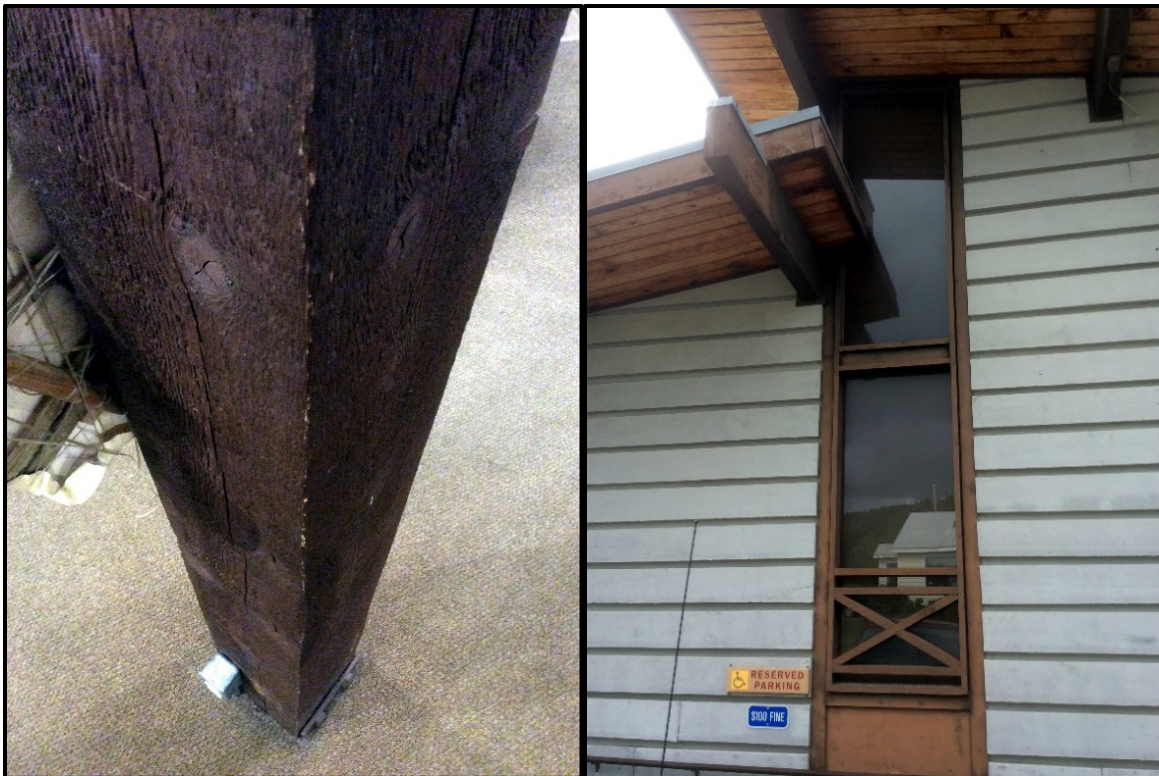
Photo 26: 8x8 rough cut post in main gallery (Left) (Cultural Alaska/Wellspring Group 2017). Photo 27: Original wire-reinforced glass windows and “X” pattern accent trim (Cultural Alaska/Wellspring Group 2017).
