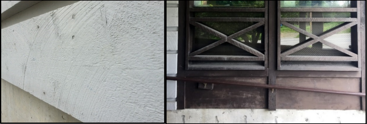
Photo 24: 2x10 siding with circular saw marks (Left) (Cultural Alaska/Wellspring Group 2017). Photo 25: “X” pattern accents on original window openings (Cultural Alaska/Wellspring Group 2017).
